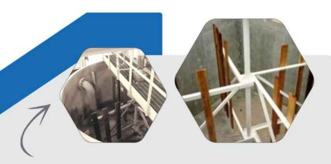
Flocculators for water and wastewater treatment plant
